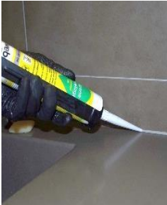
Figure 1. Sealant application
